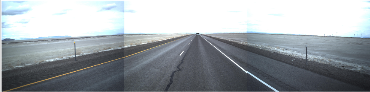
Figure 6-3: Interstate 80 in 2014 (UDOT 2015b).
