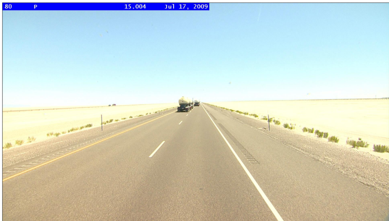
Figure 6-2: Interstate 80 in 2009 (UDOT 2015b).
